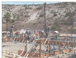
August 2004 Foundation being poured on our new home.
