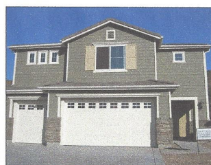
July 2005 Our rebuilt home is complete!
