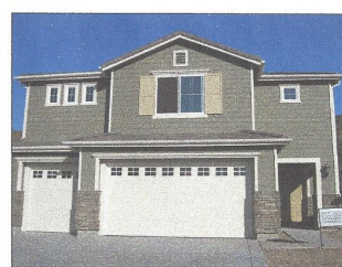
July 2005 Our rebuilt home is complete!
