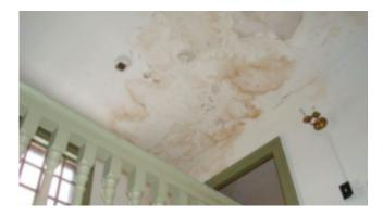
An illustration of ceiling damage due to an ice dam
