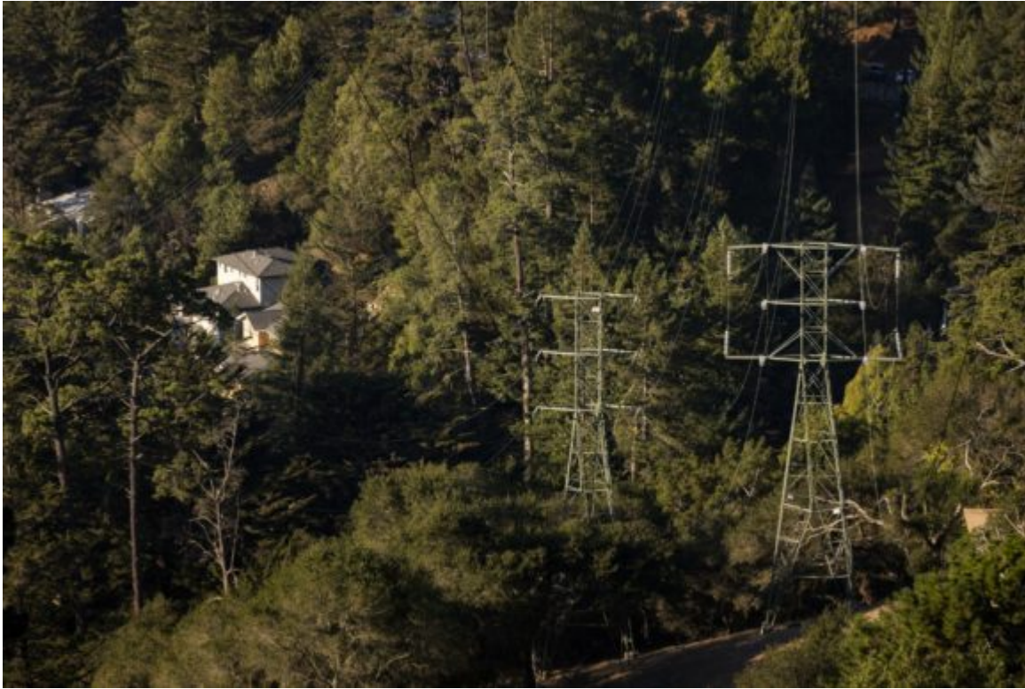
Homes sit nestled amongst dense brush and power transmission lines in the Oakland Hills area of Oakland, California, on Oct. 29, 2020. Photographer: Philip Pacheco/Bloomberg
