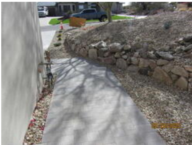
West Unit Exterior Mar 3, 2025
