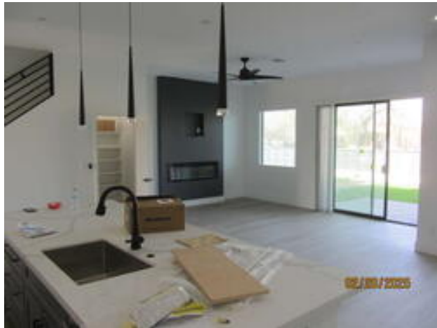
Middle Unit Interior Mar 3, 2025
