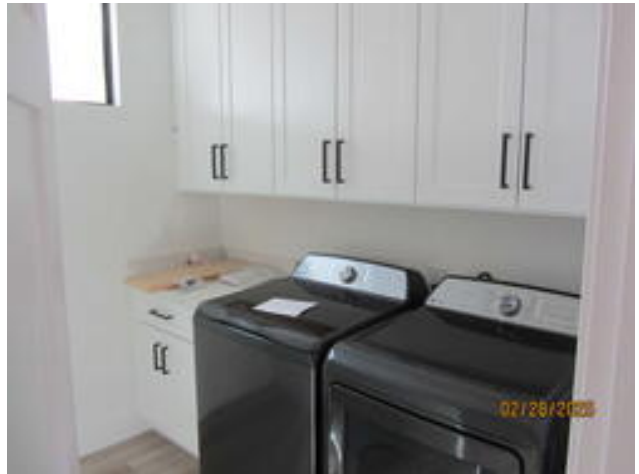
East Unit Interior Mar 3, 2025
