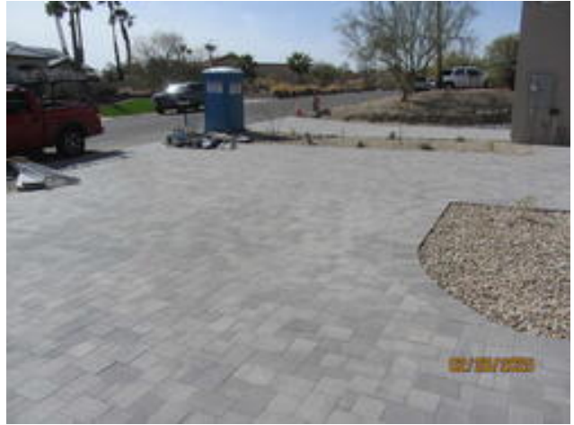
Driveway Pavers Mar 3, 2025
