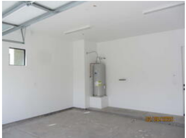
West Garage Mar 3, 2025
