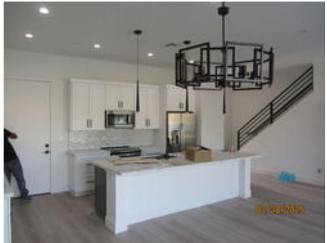
Middle Unit Interior Mar 3, 2025
