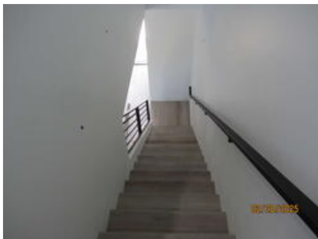
East Unit Exterior Stairs Mar 3, 2025
