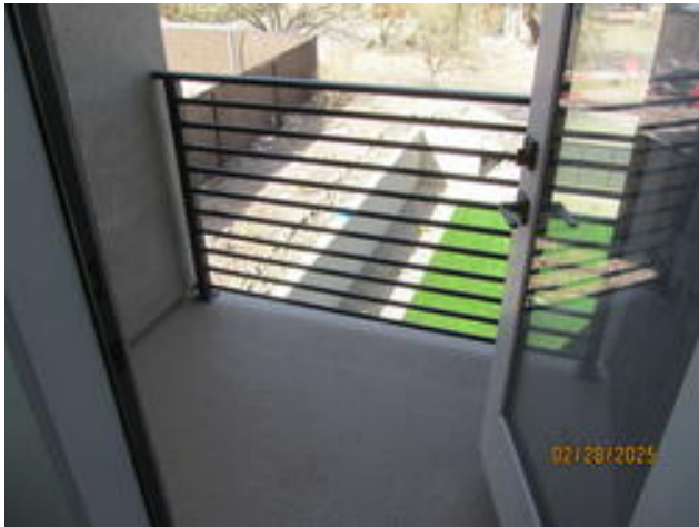
West Unit Deck Mar 3, 2025
