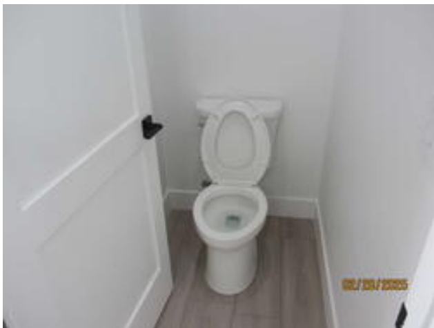
West Unit Interior Mar 3, 2025
