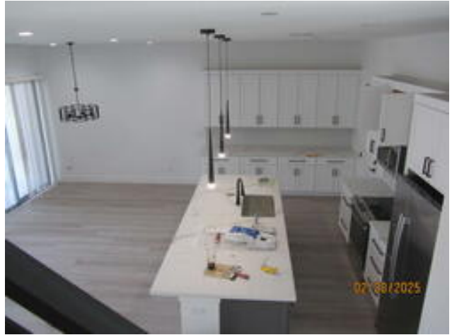
West Unit Interior Mar 3, 2025
