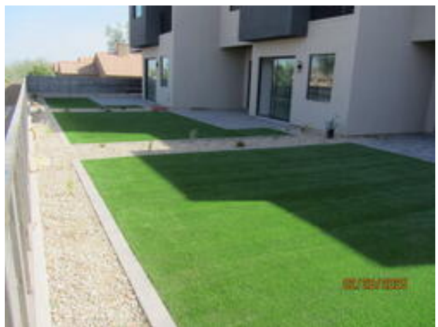
East Rear Yard Landscape Hardscape Mar 3, 2025
