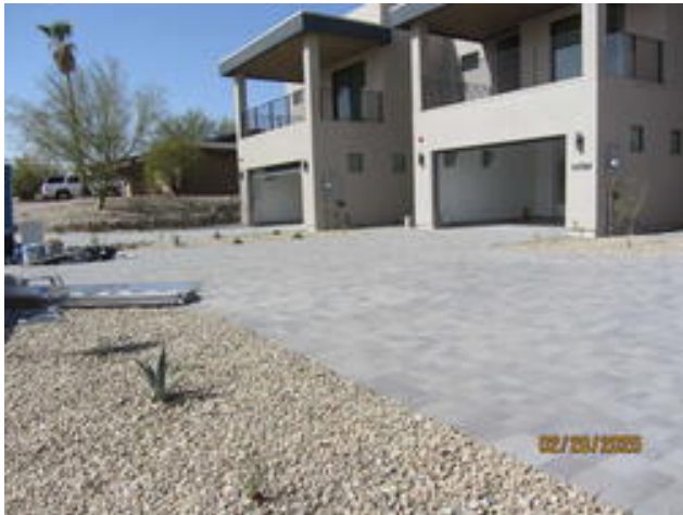
Driveway Pavers Mar 3, 2025
