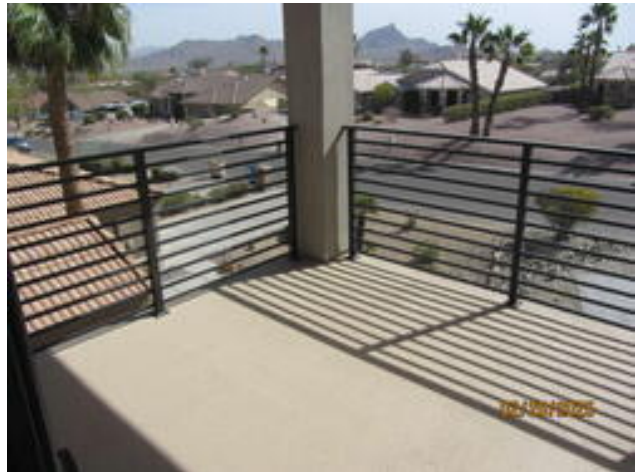
East Unit Deck Mar 3, 2025
