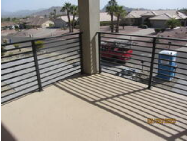
West Unit Deck Mar 3, 2025
