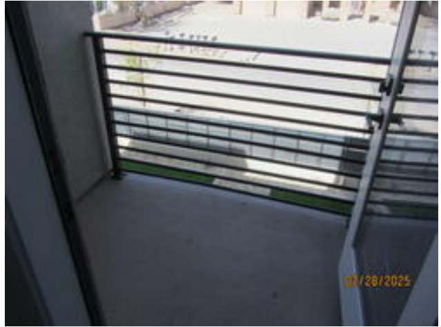
East Unit Deck Mar 3, 2025
