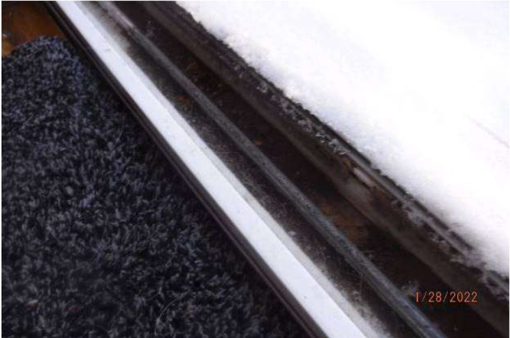
Visible soot/char/ash was observed at the base of the west sliding glass door.
