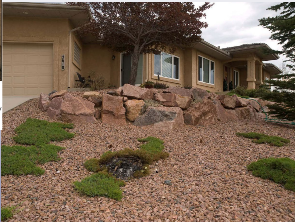
Noncombustible stucco and effective landscape management protected this house during the Carr Fire in Redding, CA in 2018. Photo: FEMA
