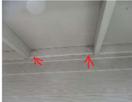
Bird Blocking Installed With Splintered Material
