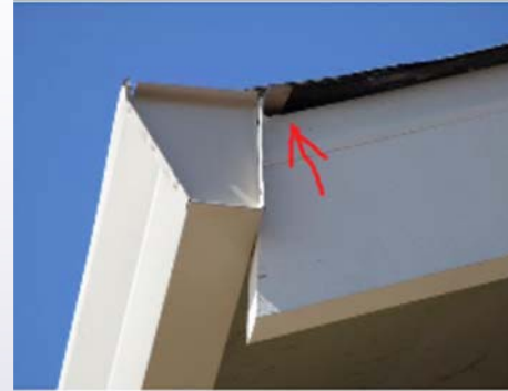
Side View Of Composite Roofing Raised Up Because Of Improper Gutter Install
