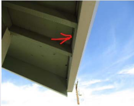
Roof Sheathing Is Not Cut Properly At End Of Roof Truss Ends
