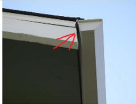
Roof Truss Ends Not Cut Square At Same Distance
